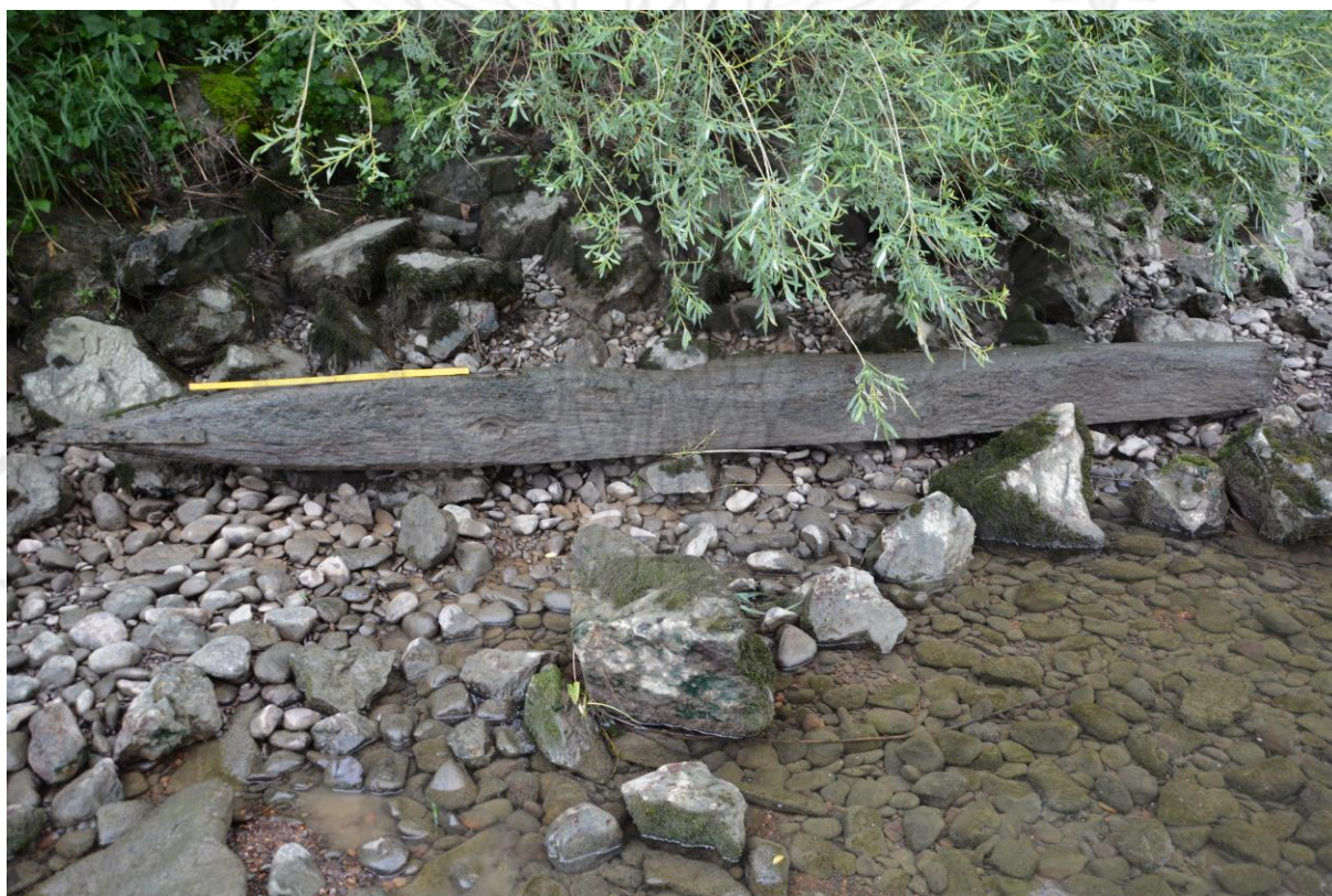
Fig. 6 – Piles with iron forged reinforcement on the bank of the Váh River (photo by: K. Daňová)
